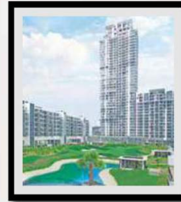
M3M golfstate Fairway GOLF COURSE ROAD EXTENSION SECTOR-65, GURUGRAM
